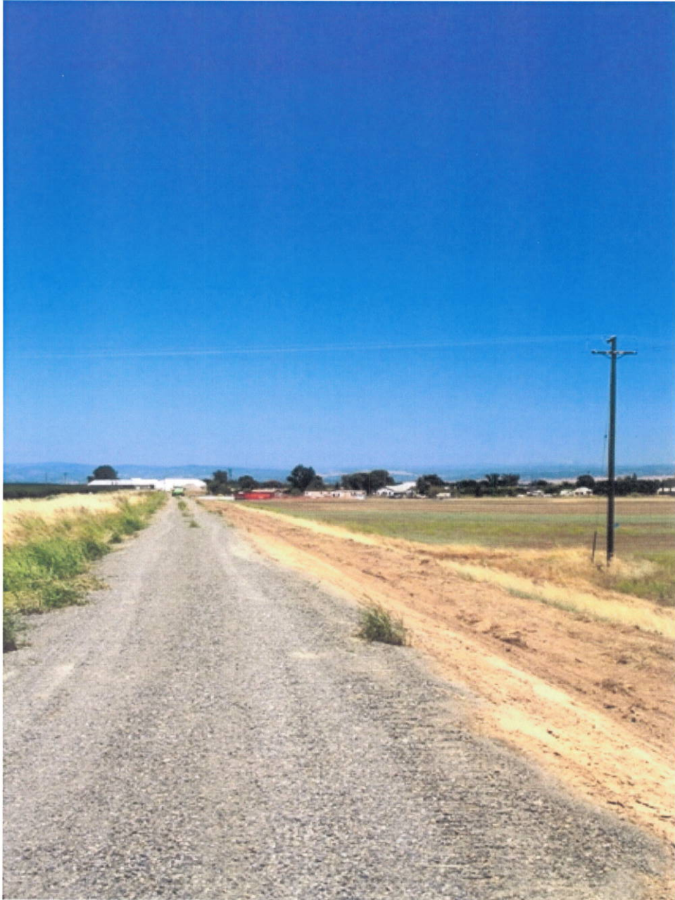
Station 146+08 Looking East
