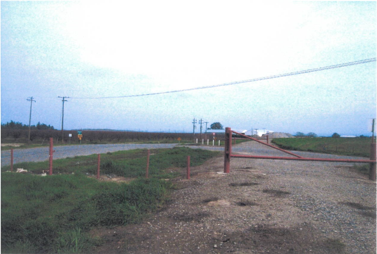
Station 164+37 Looking East Waterside
