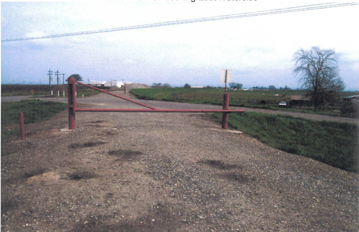
Station 164+37 Looking East Landside
